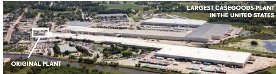
Arcadia, WI: Est. in 1970 with 35,000 sq. ft. 3,053,345 sq. ft. | 283,665 sq. mt. | 70 acres under roof
