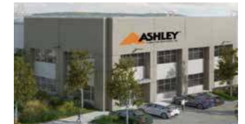
Spanaway, WA: Opening in 2021 1,336,673 sq. ft. | 124,181 sq. mt. | 31 acres under roof
